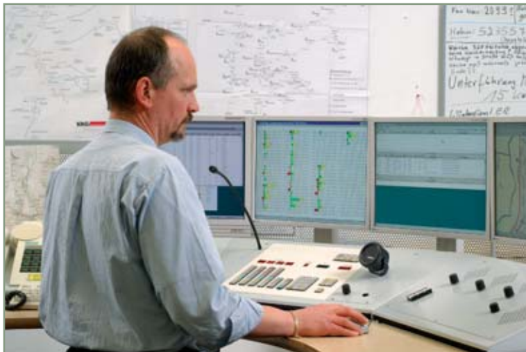
> MOBILE-ITCS allows dispatchers to control radio communication out of the ITCS.
