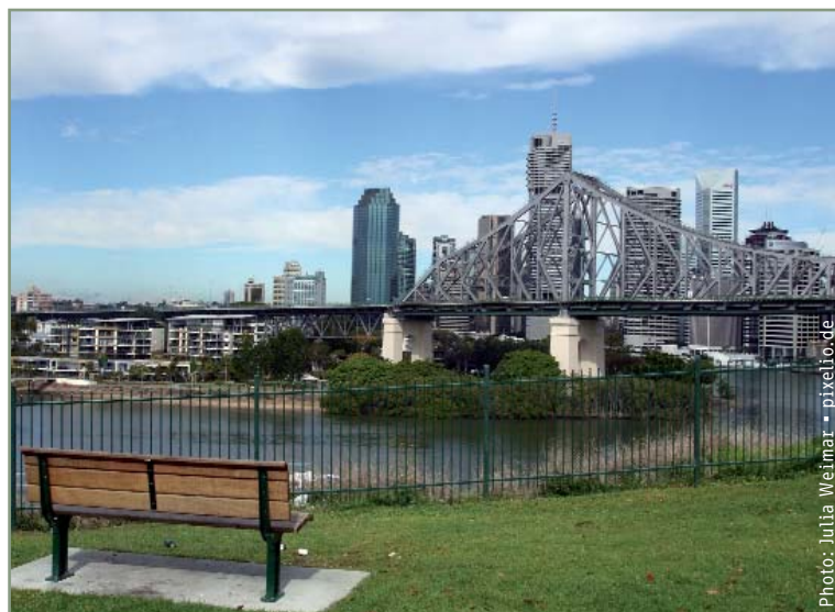
> Customer First Project: Brisbane strives for reliable service and real-time passenger information.
